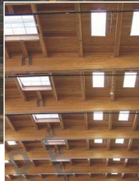
Interior View of Heavy Timber Roof.
